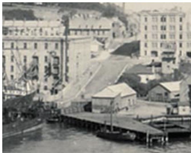
Cart ramps ran up the steep slopes from the Bay in 1904.
